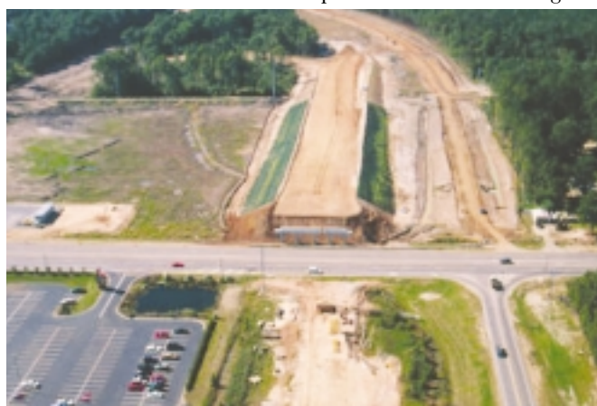
WEB BID The e-bid was $14 million for this Georgia highway job.
